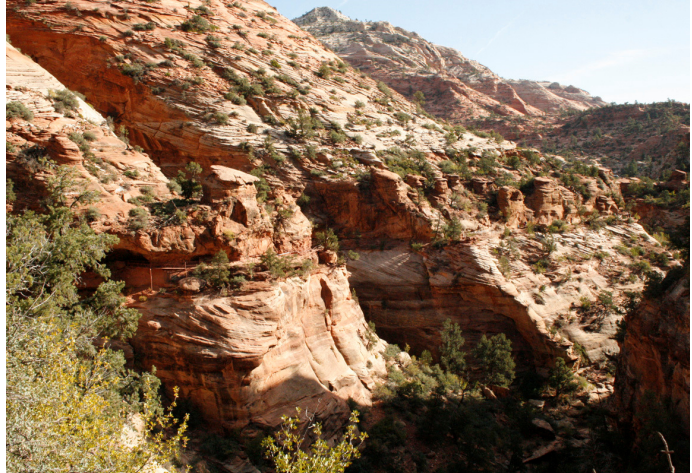
Viewpoint Trail – The Overlook Trail. The trail follows the base of the red rocks. The catwalk can be seen at the middle left of the photo where it swings out, then under the rocks.
