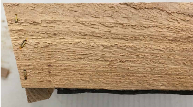
Angled Sides (Side View) – Sides of box showing the canted side and end piece extending down to act as a foot. Stapled screen is also visible.
