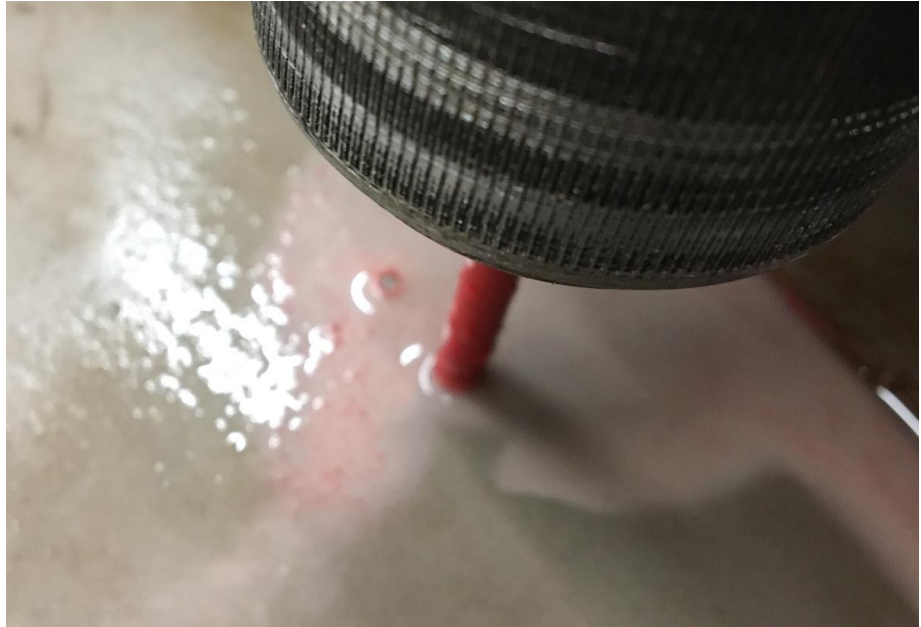
Drilling in progress
